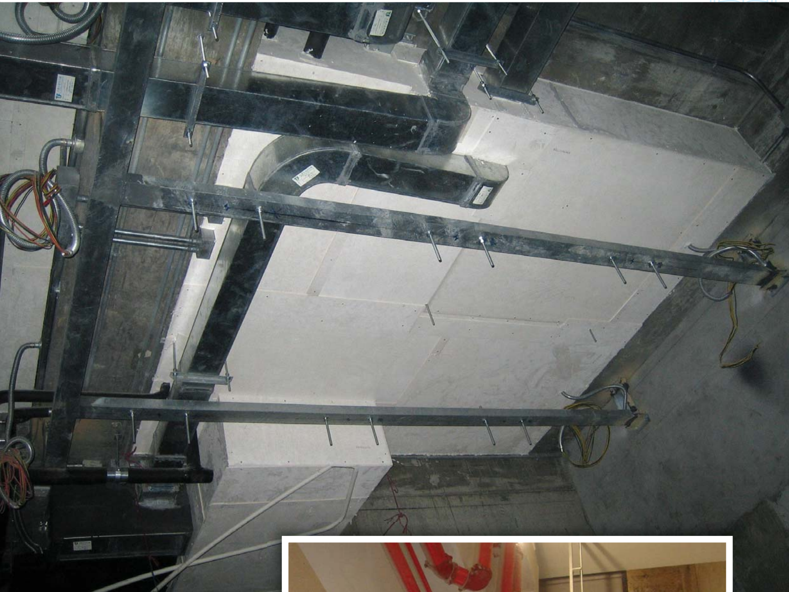
General M&E services enclosure (clockwise from top): PROMATECT®-H for the carpark of Tseung Kwan O residential building in Sai Kung District, New Territories, Hong Kong; VICULCAD® at the basement of Vivocity Singapore; PROMATECT®-H for outside of a warehouse at 9 Benoi Sector, Singapore.
