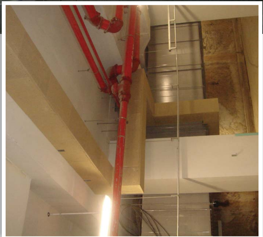
General M&E services enclosure (clockwise from top): PROMATECT®-H for the carpark of Tseung Kwan O residential building in Sai Kung District, New Territories, Hong Kong; VICULCAD® at the basement of Vivocity Singapore; PROMATECT®-H for outside of a warehouse at 9 Benoi Sector, Singapore.
