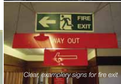
Fire exit at the side entrance of a residence building
