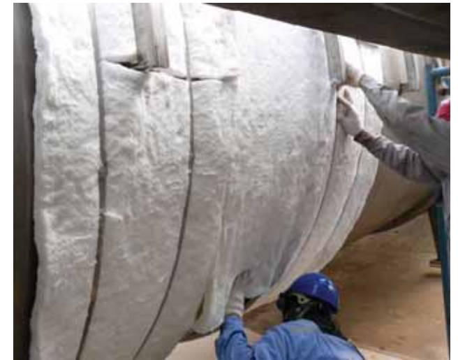
Promat ALSIFLEX®-1260 ceramic fibre mats were installed at an on-shore yard prior to shipping to the Erawan Riser Platform.
