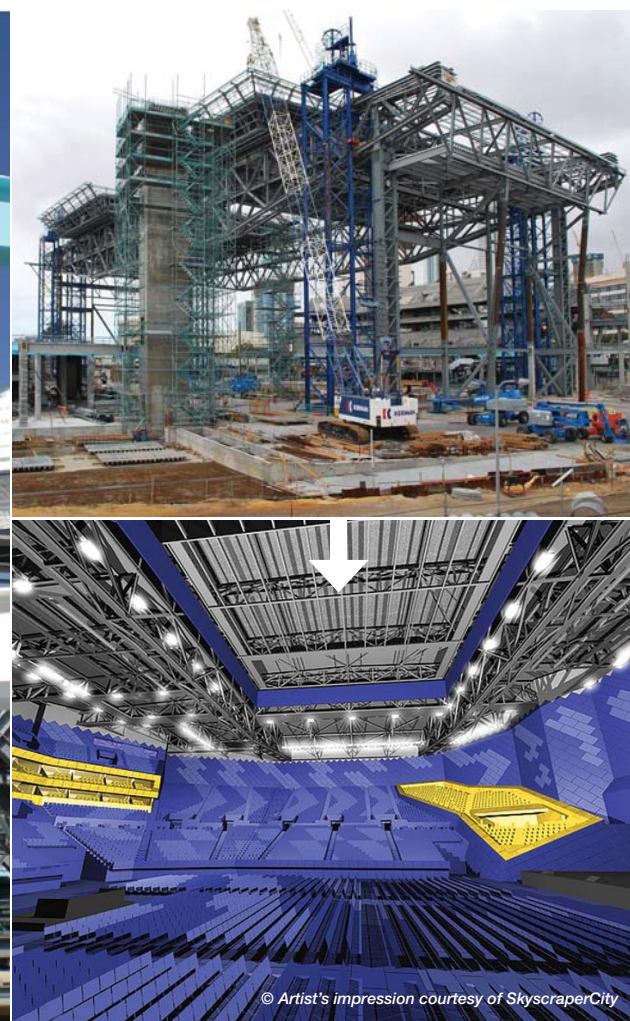
Caico SPRAYFILM® WB3 applied with brush and roller for touch up after sprayed onto the steel structure
