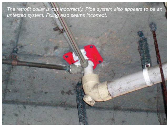
Incorrect collar size and installation! Collar seems altered and fixing appears incorrect.
