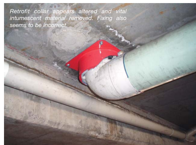
Pipe not completely and securely surrounded by retrofit collar (below). Installation of PROMASTOP UniCollar (right) appears incorrectly and inappropriately cut away.
