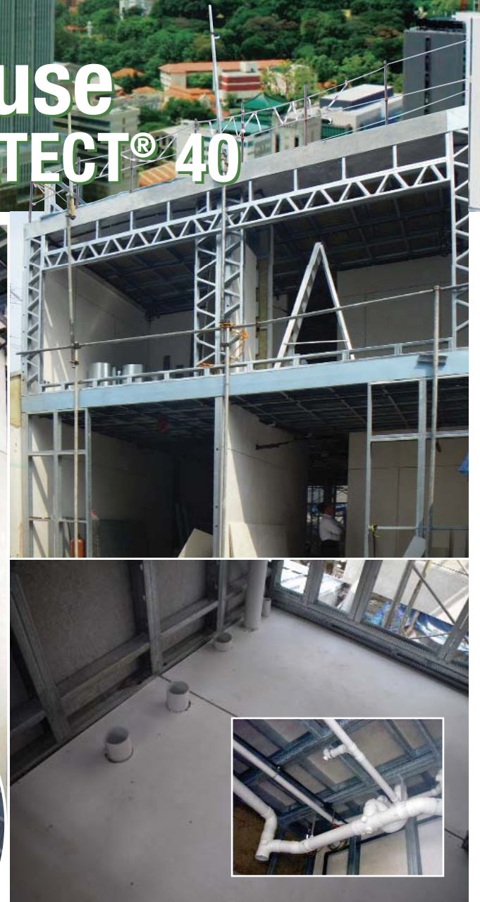
(Clockwise from above left) A robust, impact resistant enclosure to the stairwell is ensured with a wall constructed from PROMATECT® 40 boards; the basic skeletal of the house structure in progress; 25mm PROMATECT® 40 floating floor in the bathroom prior to waterproofing, the sanitary pipes are neatly concealed (inset) and the fire resistant pipe collars can be introduced with ease.
