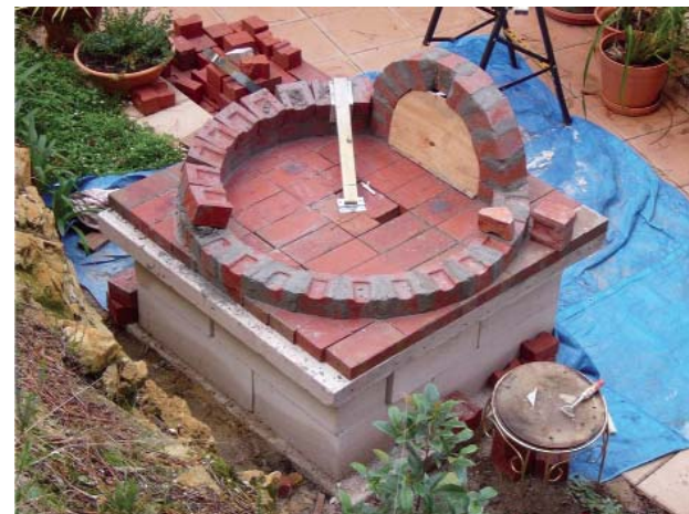
PROMASIL® 1000 should be applied on top of the "circled" brick work/concrete area, including underneath the first preceding layer of the brick/concrete forms.
