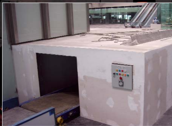
120 minute fire resistant enclosure made of PROMATECT®-H boards secured to steel framework.
