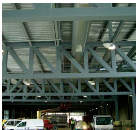
Adelaide Bus Station, with structural steel protected
