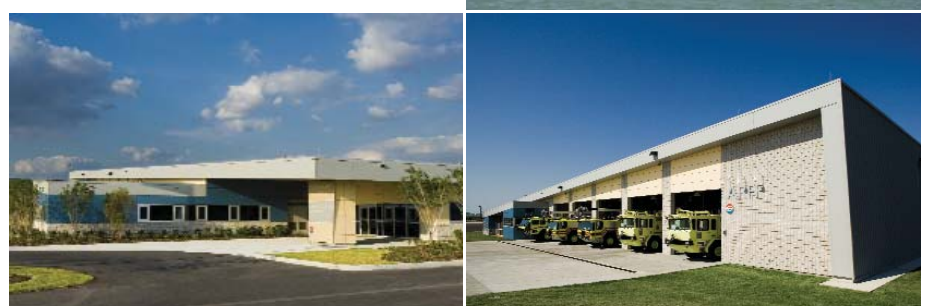
The Airport Rescue and Fire Fighting Facility at Hong Kong International Airport (right) and Tampa International Airport in Florida (below).
