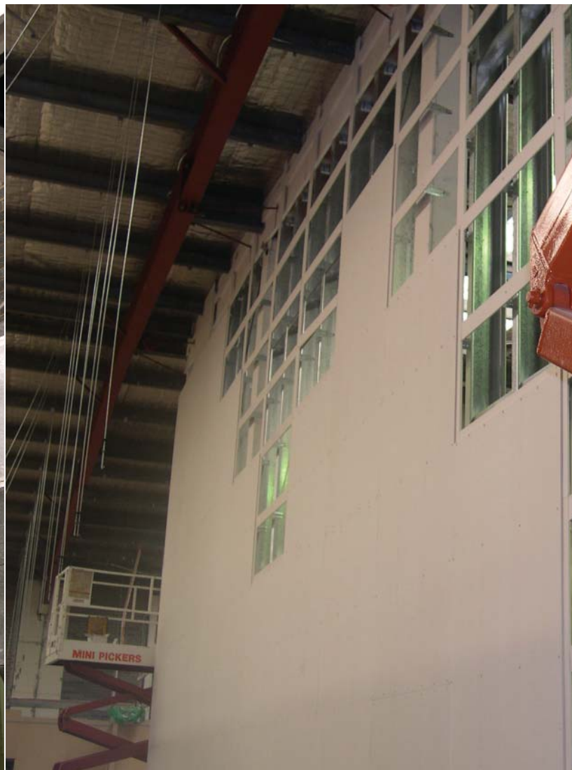
9mm PROMATECT®-H cover strips and sheets installation on the first side of the 90 minutes wall in Alexandria, Sydney Warehouse.
