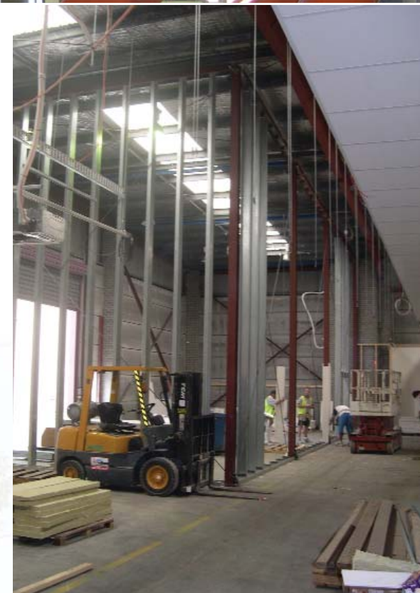
Below: Steel erected for the 90 minutes wall. It is important to note that structural steel within the wall cavity is clad separately.
