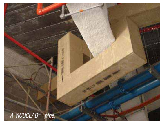
HVAC ducts after cladding with PROMATECT®-H.
