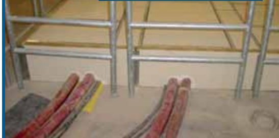
Cable entries penetrate the PROMAVIC® panels.
