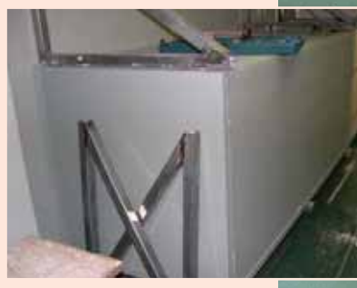
(Right and top right) PROMATECT® -L500 two hours fire rated self-supporting ducts in Telstra Exchange of City North, Sydney, Australia.
