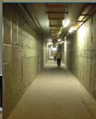
Four hours PROMATECT®-H partitions flanked on both sides of the wall; (inset) before completion of final layer boards.
