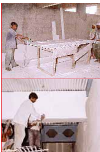
The asbestos-free PROMATECT® 250 boards are also easy to work with and install.
