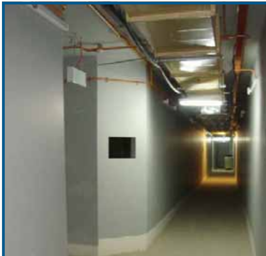
Four hours PROMATECT®-H partitions flanked on both sides of the wall; (inset) before completion of final layer boards.
