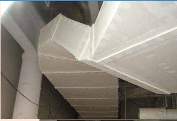
(Top right, below and here) PROMATECT® -H two hours fire rated post cladding steel ducts in Queensway Fire Station, Singapore.
