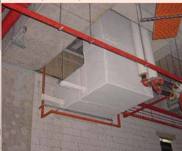
(Left, top, below and far left) PROMATECT® -H fire rated ductwork systems throughout the Changi Water Reclamation Plant.
