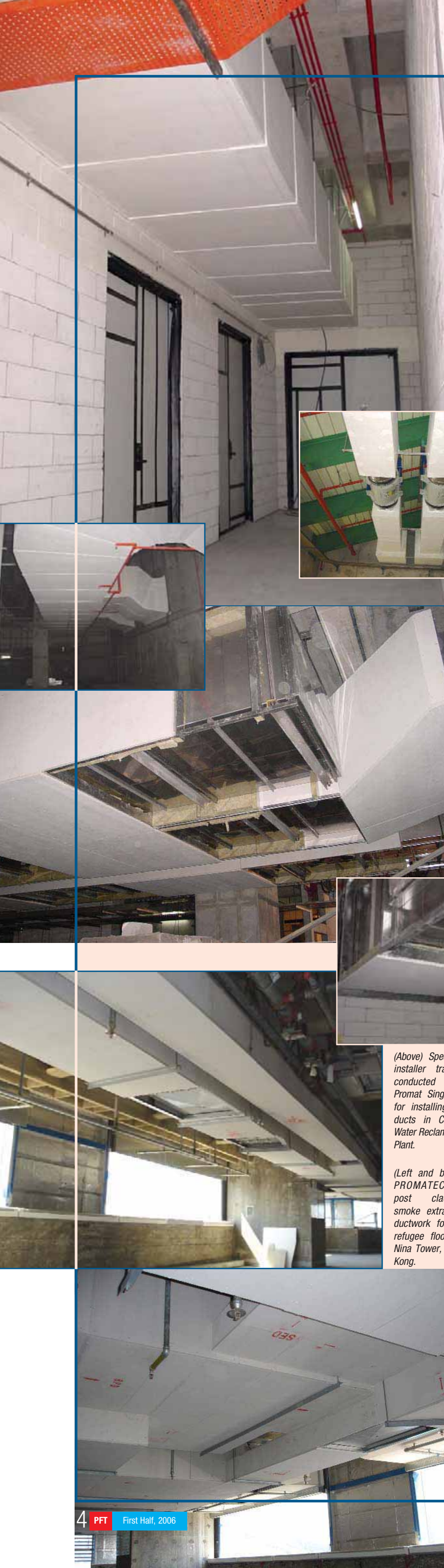
(Left, top, below and far left) PROMATECT® -H fire rated ductwork systems throughout the Changi Water Reclamation Plant.
