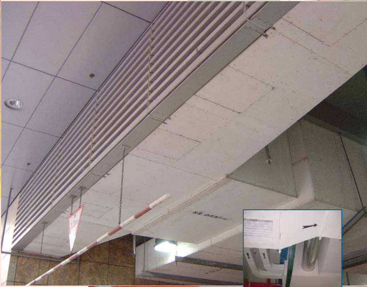
(Bottom) PROMATECT® -H post cladding smoke extraction ductwork in Langham Place, Hong Kong.
