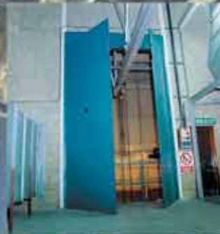
Industrial strength fire door for maintenance hangars
