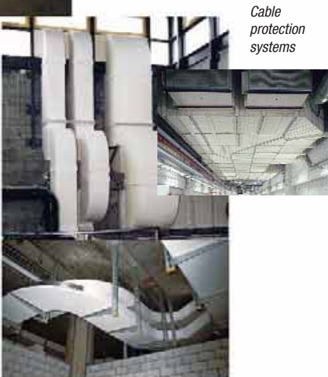
Fire resistant kitchen smoke extraction ducts
