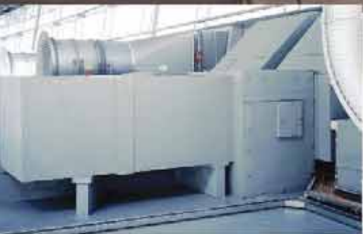
Structural steelwork protection using PROMAPAIN ® systems, air conditioning and smoke extraction ductwork systems in airport terminals
