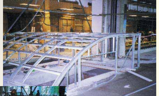
Skeletal frame construction of the baggage entry compartment.
