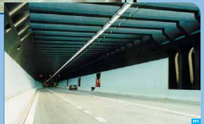
Right: Kennedy Tunnel, Antwerp, Belgium
