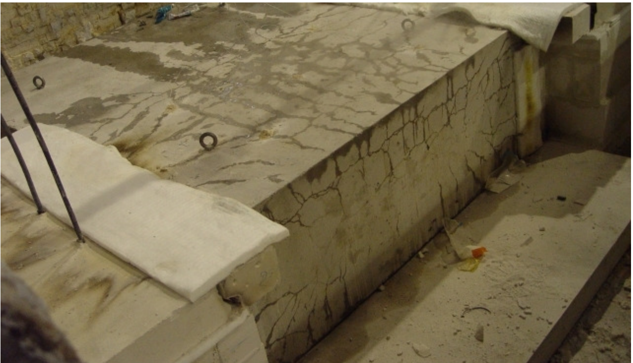
A photograph from a reverse angle showing the side wall during cooling down. It can now clearly be seen that beside the radial pattern, a single longitudinal crack dominates.
