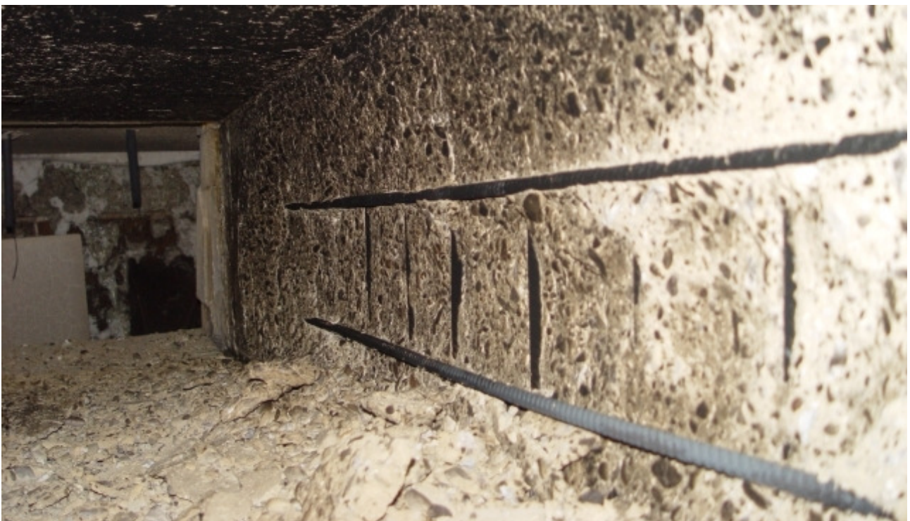
The inside of the heated tunnel tube a few days after testing, showing that the reinforcement has been laid bare.
